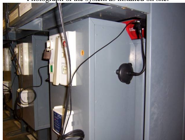
Photograph showing ultrasonic sensor pointed at the circuit breaker spouts
